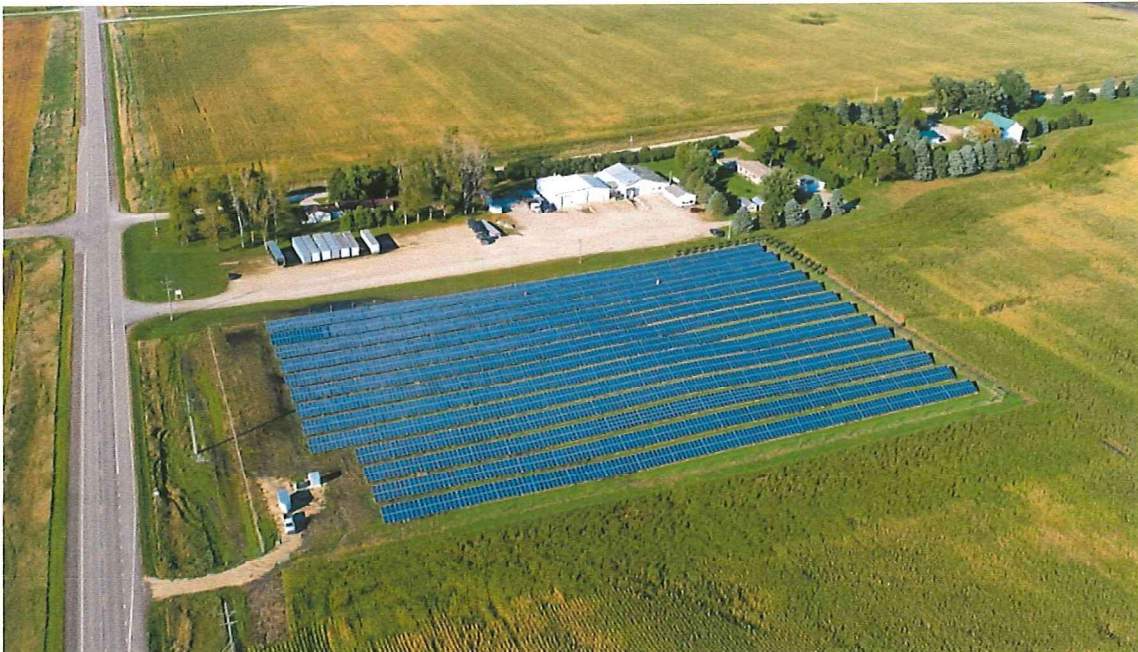
1MW CSG in Waseca County
