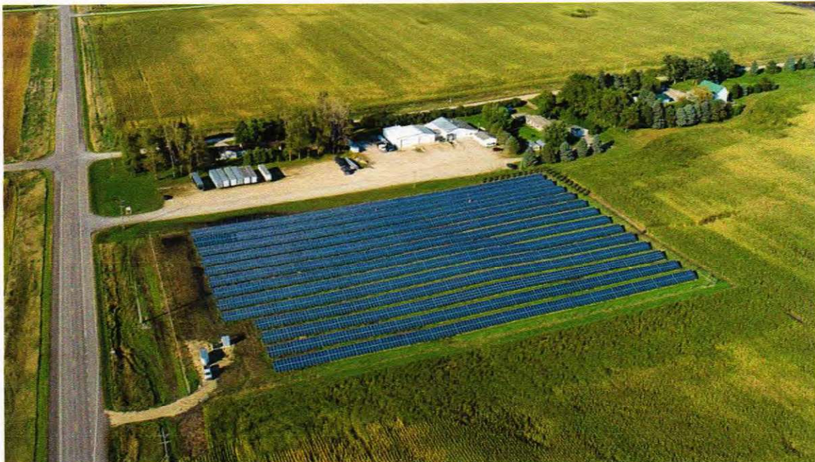
1MW CSG in Waseca County
