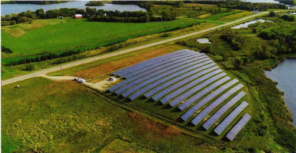
1MW CSG in Pope County
