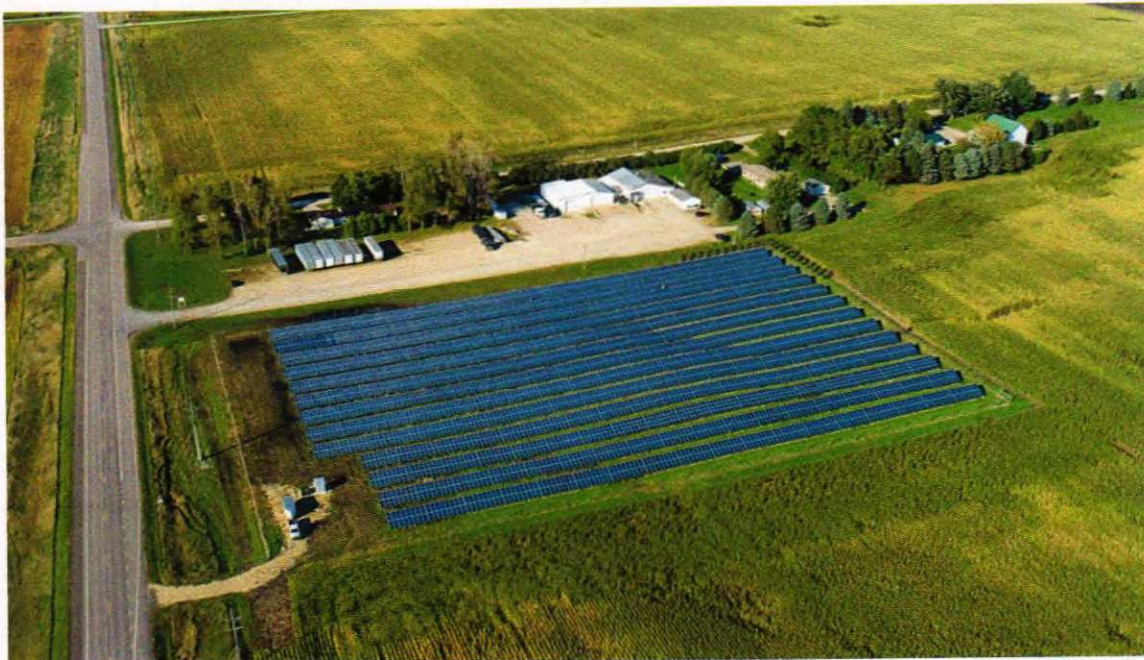
1MW CSG in Waseca County
