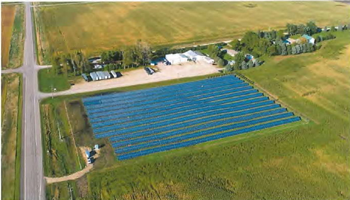
1MW CSG in Waseca County
