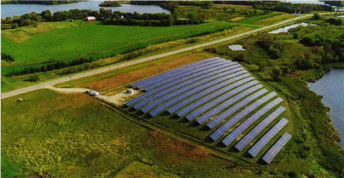
1MW CSG in Pope County
