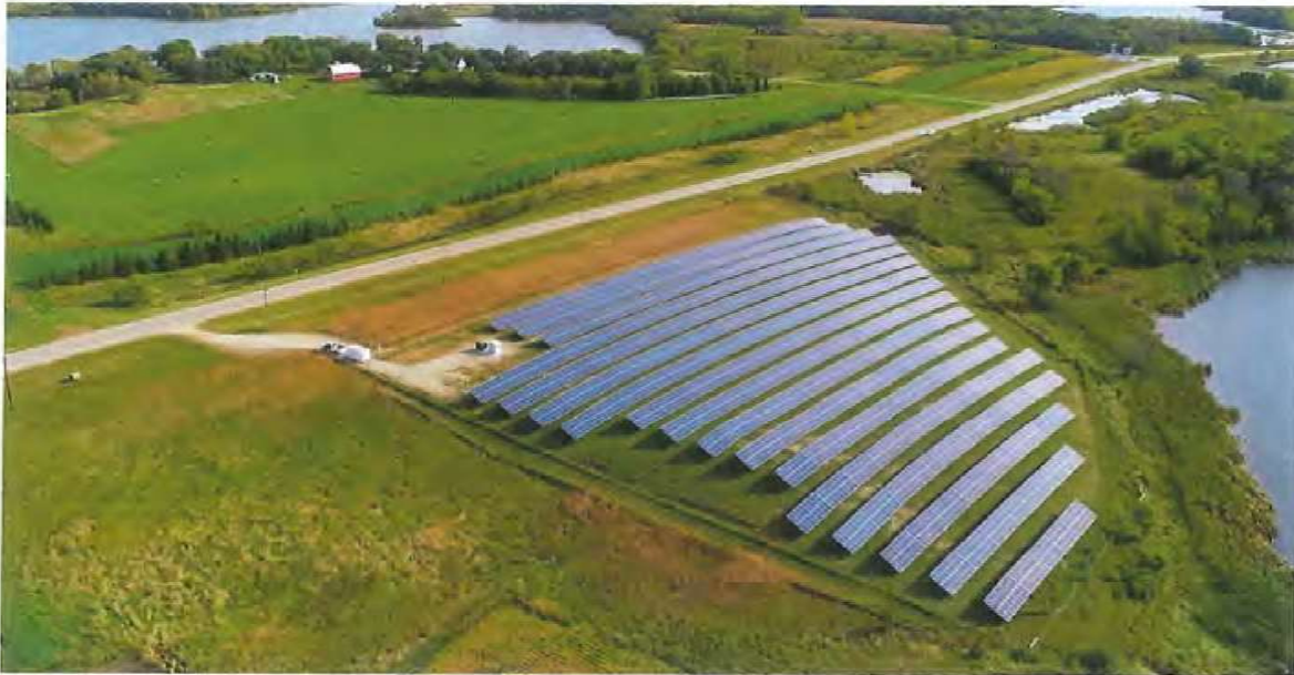
1MW CSG in Pope County
