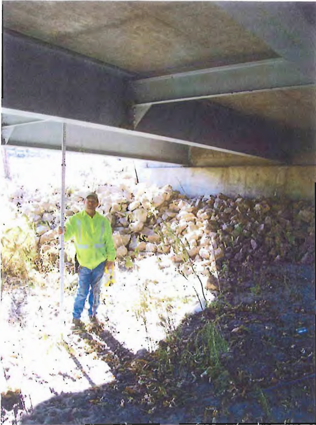
Underneath westbound bridge location near trial showing 10' clearance standing 25' from support pillars
