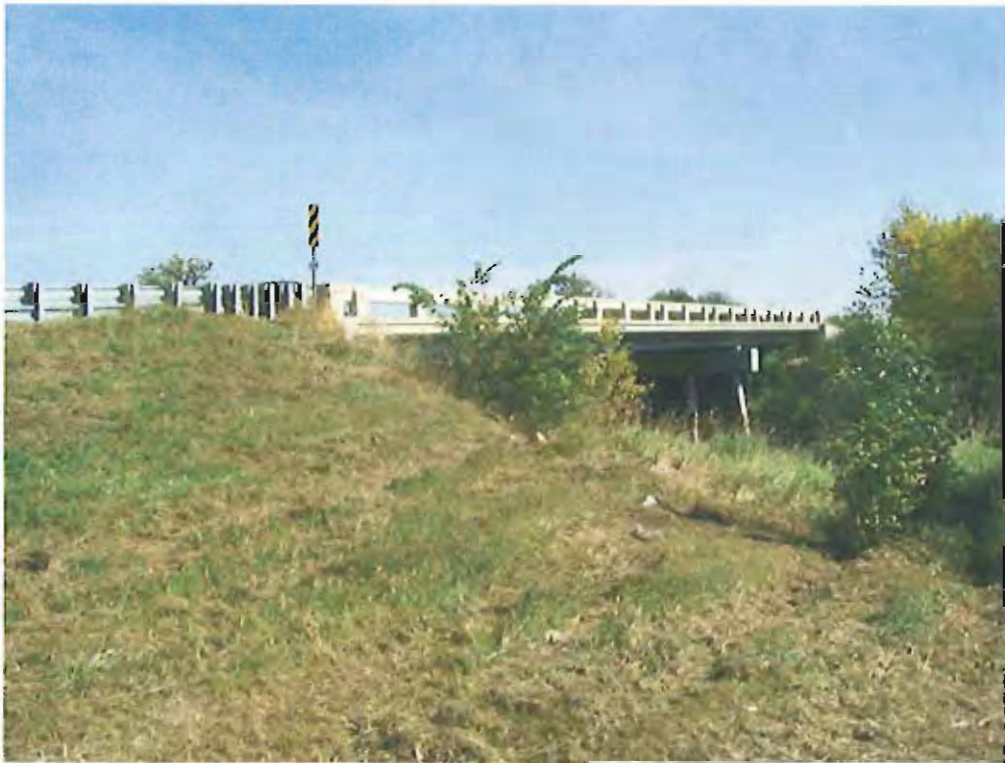
Eastbound right-of-way of US Hwy 212 looking east approaching Buffalo Creek overpass bridge
