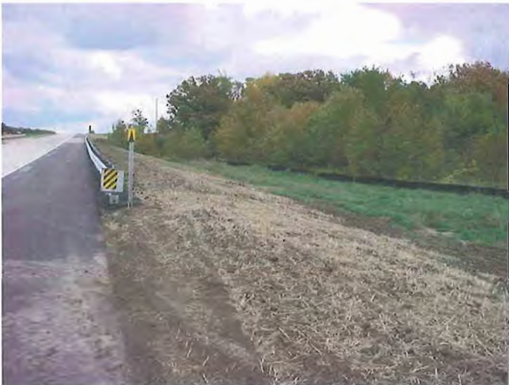
Eastbound right-of-way of US Hwy 212 looking east approaching Buffalo Creek overpass bridge
